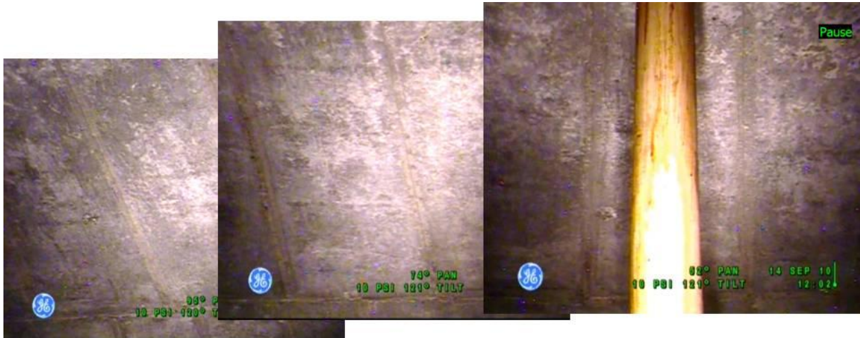
Figure 12-2: Compilation of Photographs of Tank 241-S-103Dome
