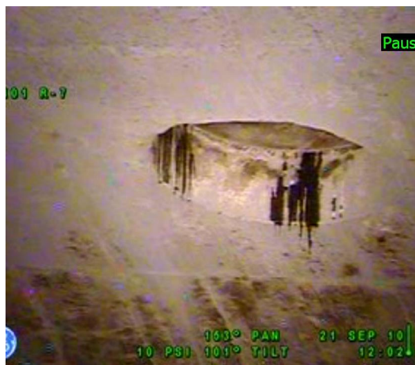
Figure 11-1: Tank 241-S-101 Concrete Dome
