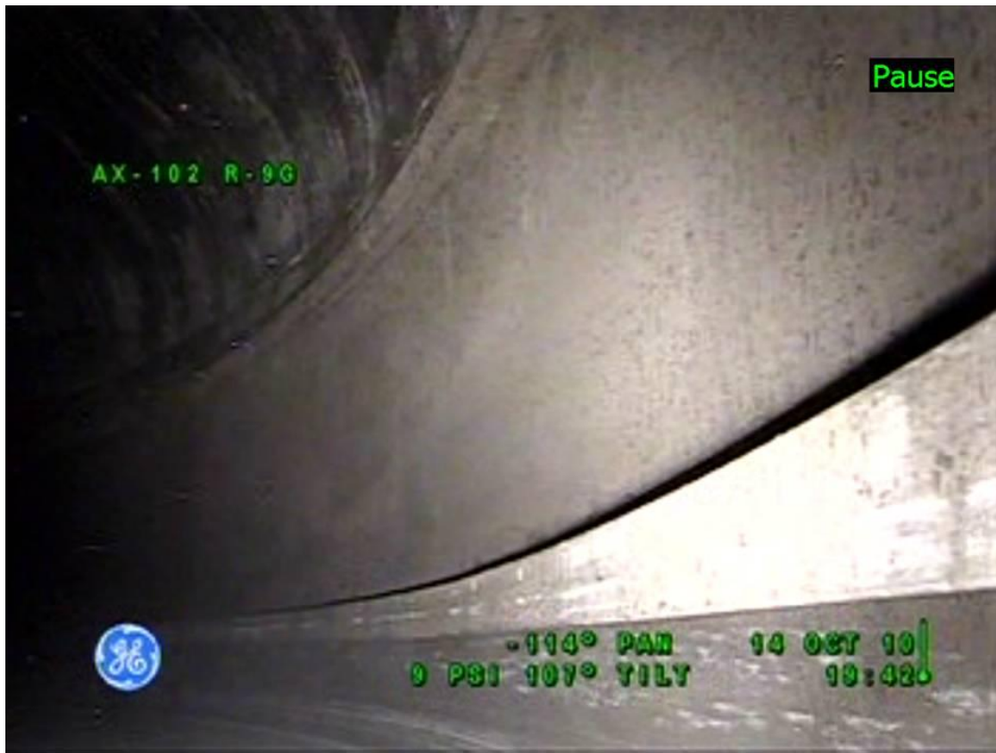
Figure 7-4: Tank 241-AX-102 Steel Liner
