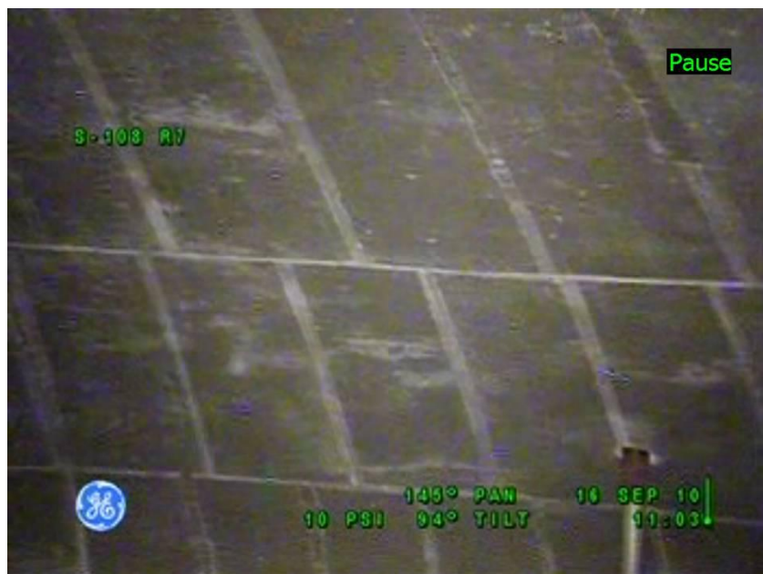
Figure 14-1: Tank 241-S-108 Concrete Dome
