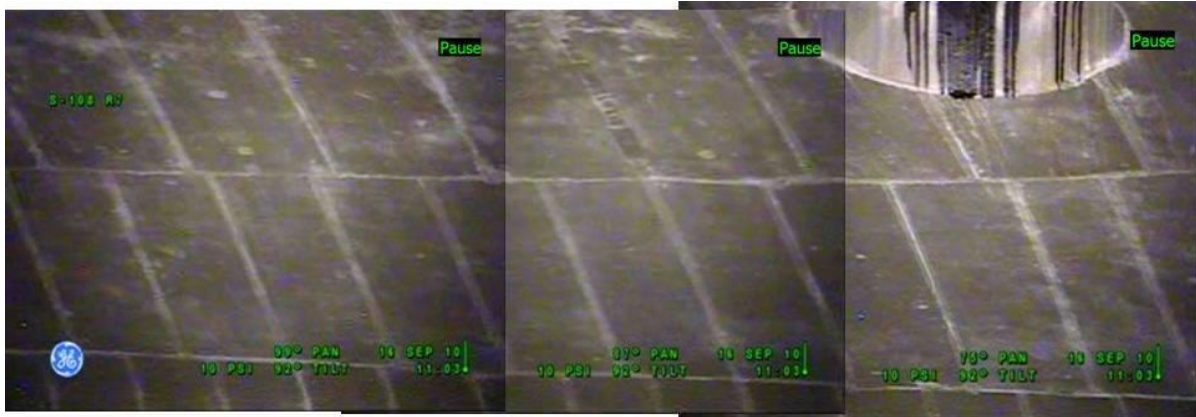
Figure 14-2: Compilation of Photographs of Tank 241-S-108 Dome
