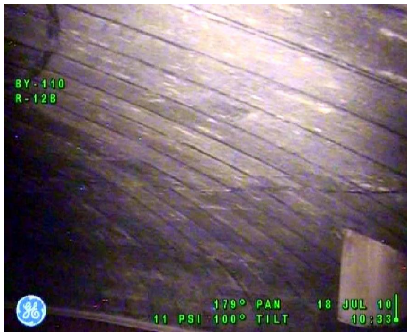
Figure 9-1: Tank 241-BY-110 Concrete Dome
