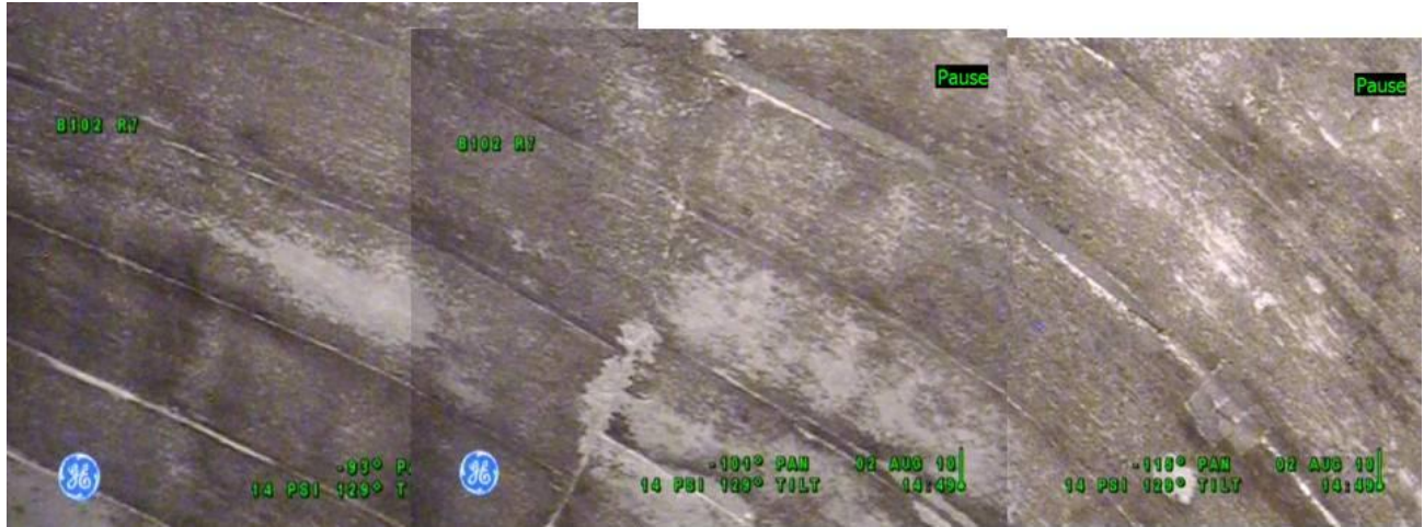
Figure 8-2: Compilation of Photographs of Tank 241-B-102 Dome
