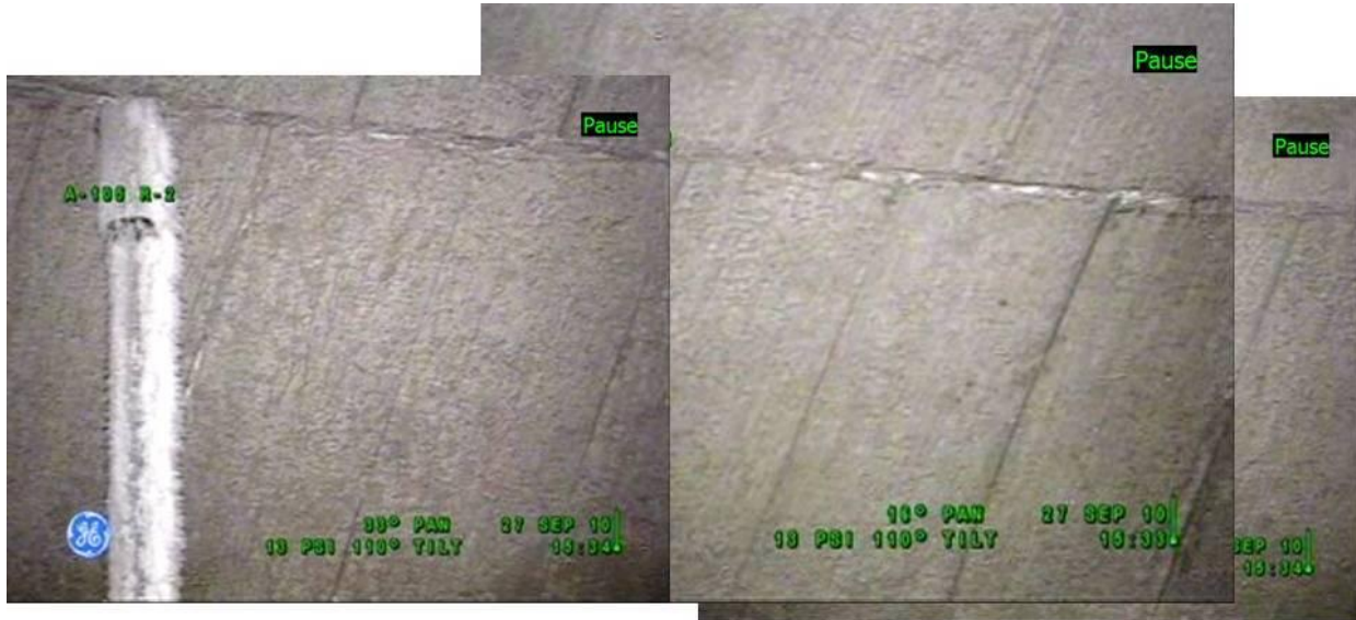
Figure 5-2: Compilation of Photographs of Tank 241-A-105 Dome
