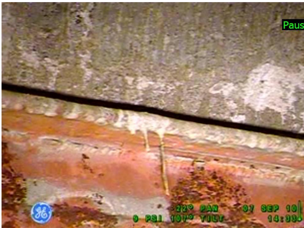
Figure 10-3: Tank 241-C-110 Steel Liner
