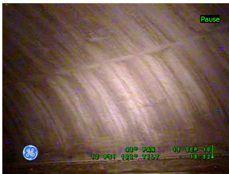
Figure 15-1: Tank 241-SX-101 Concrete Dome
