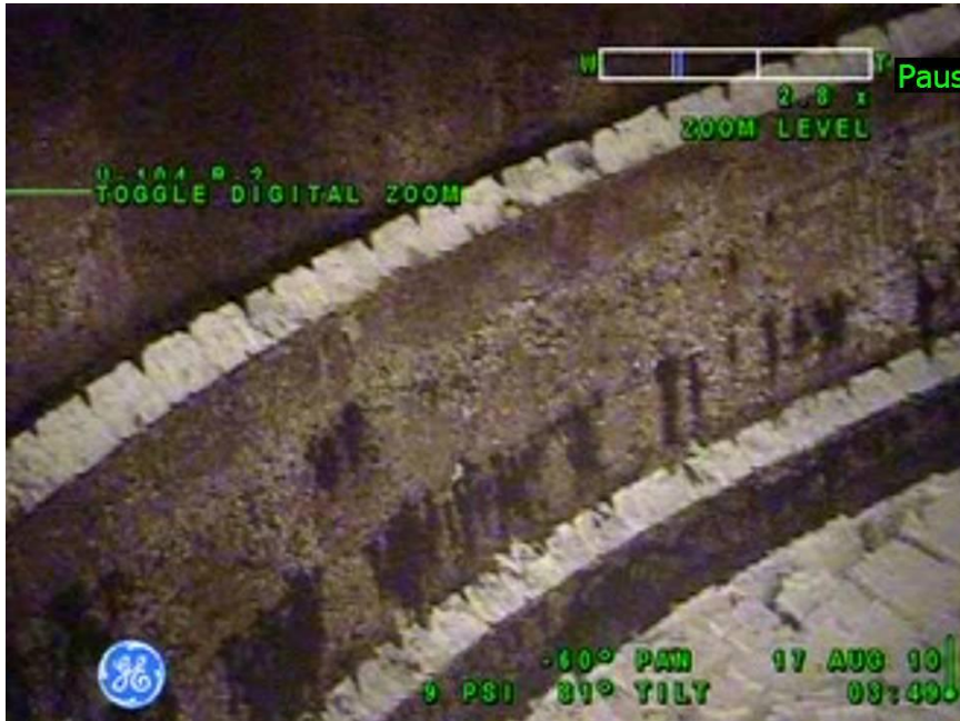
Figure 16-5: Tank 241-U-104 Steel Liner
