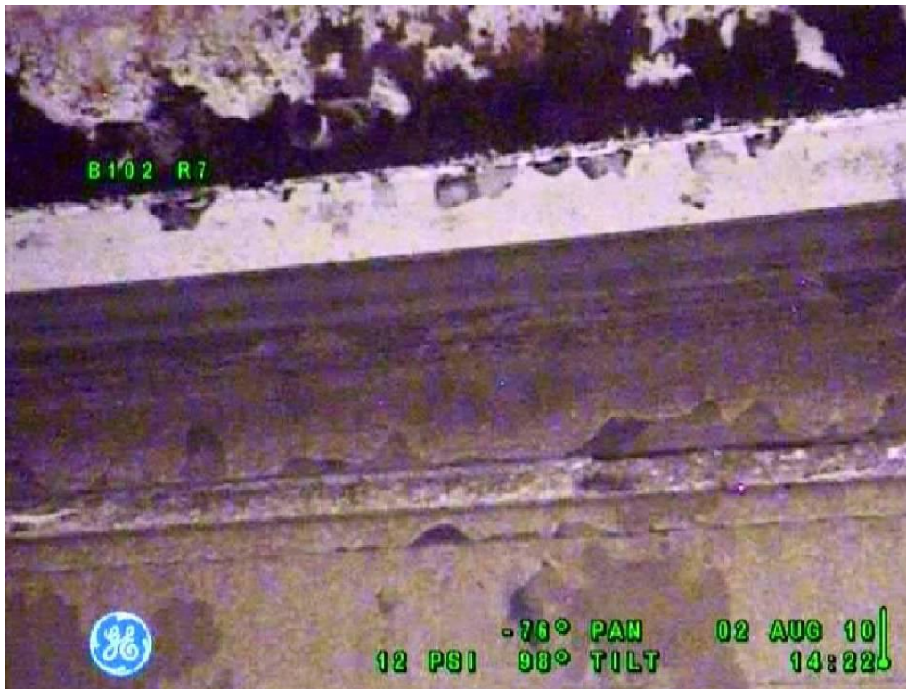
Figure 8-3: Tank 241-B-102 Steel Liner
