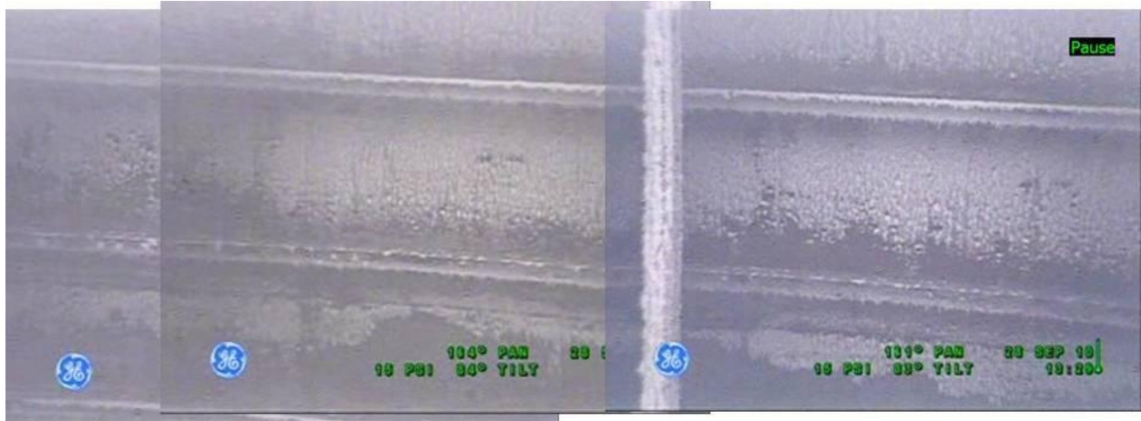
Figure 5-5: Compilation of Photographs of Tank 241-A-105 Steel Liner
