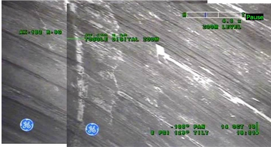
Figure 7-2: Compilation of Photographs of Tank 241-AX-102 Dome
