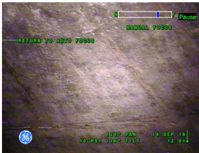
Figure 12-1: Tank 241-S-103 Concrete Dome
