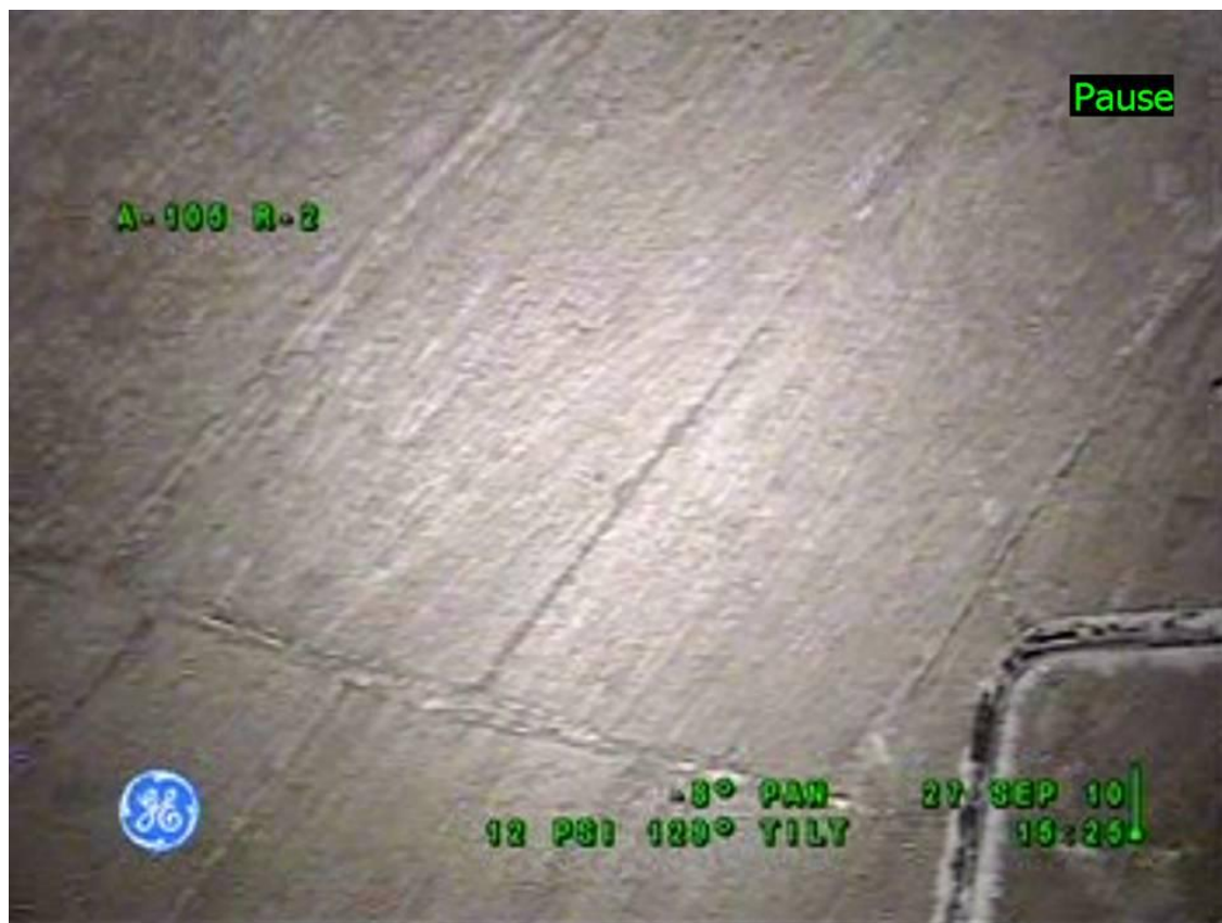
Figure 5-1: Tank 241-A-105 Concrete Dome
