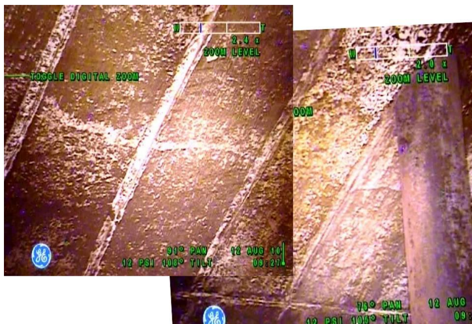
Figure 6-2: Compilation of Photographs of Tank 241-A-106 Dome
