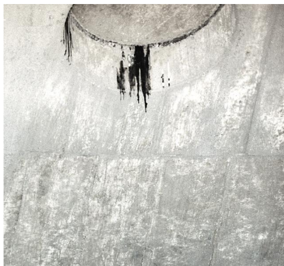
Figure 11-2: Prior photo of Tank 241-S-101 10
