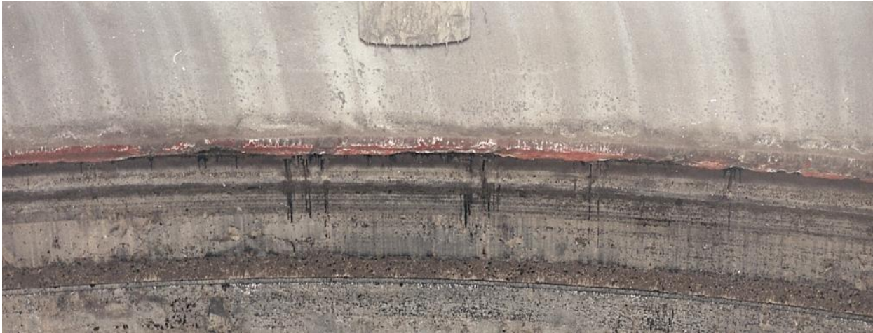
Figure 13-4: Tank 241-S-104 13 in 1984
