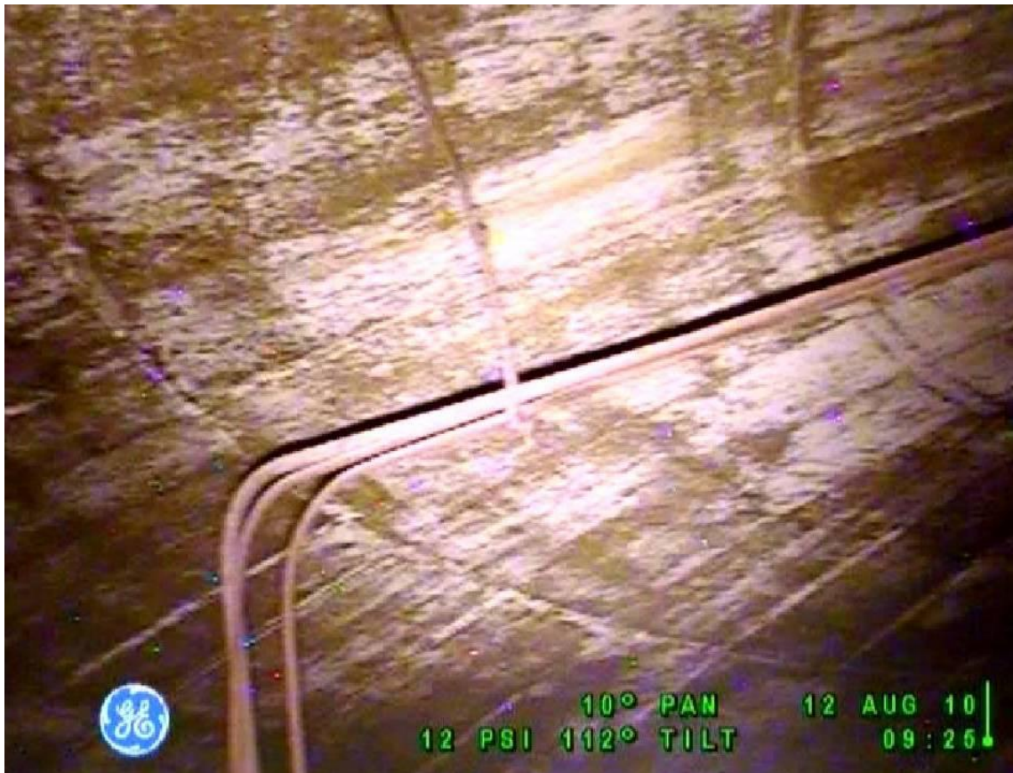
Figure 6-1: Tank 241-A-106 Concrete Dome
