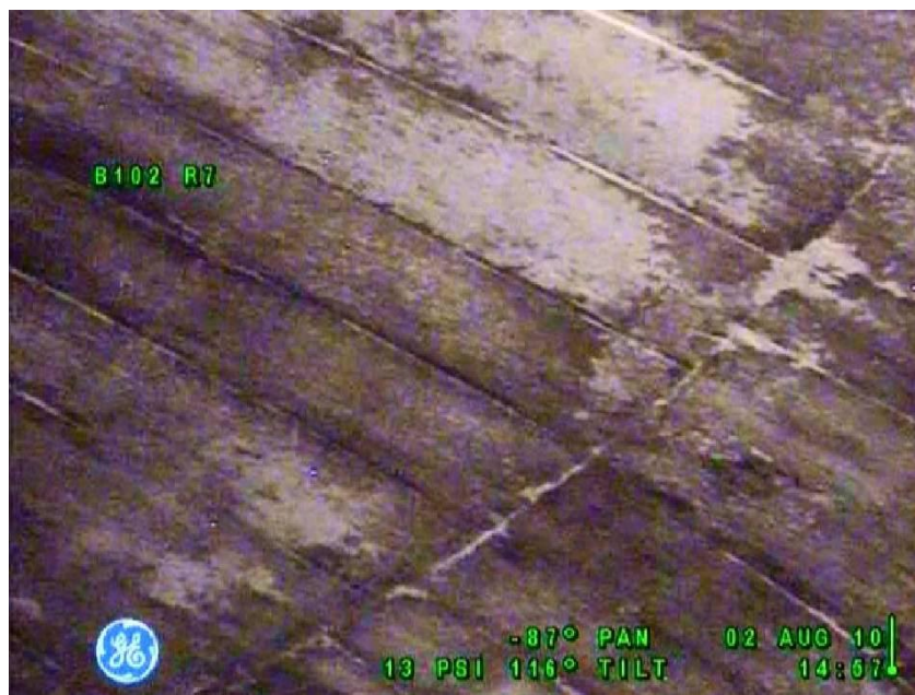
Figure 8-1: Tank 241-B-102 Concrete Dome
