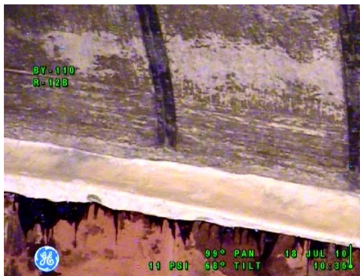
Figure 9-5: Tank 241-BY-110 Steel Liner
