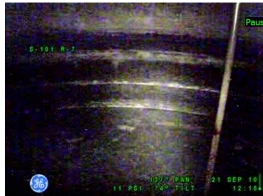
Figure 11-5: Tank 241-S-101 Steel Liner
