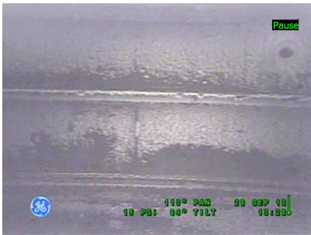
Figure 5-4: Tank 241-A-105 Steel Liner
