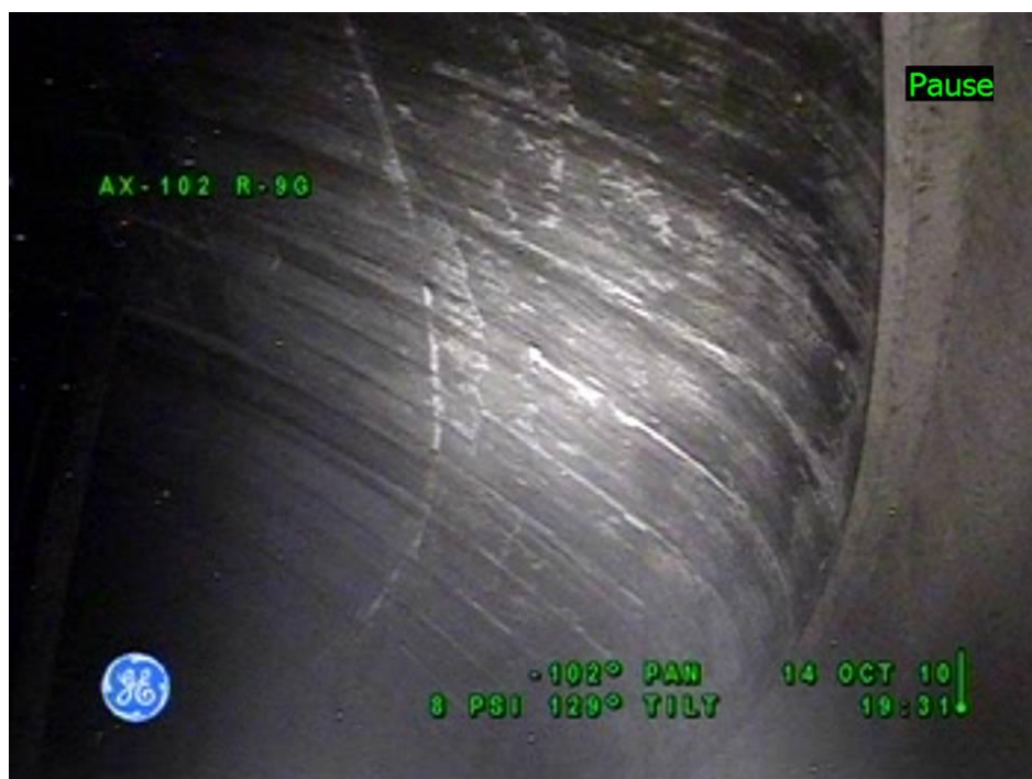
Figure 7-1: Tank 241-AX-102 Concrete Dome
