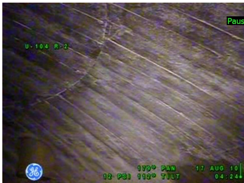
Figure 16-1: Tank 241-U-104 Concrete Dome
