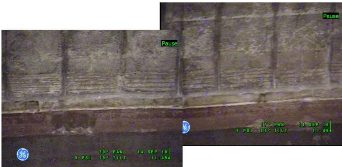
Figure 12-6: Compilation of Photographs of Steel Liner Tank 241-S-103
