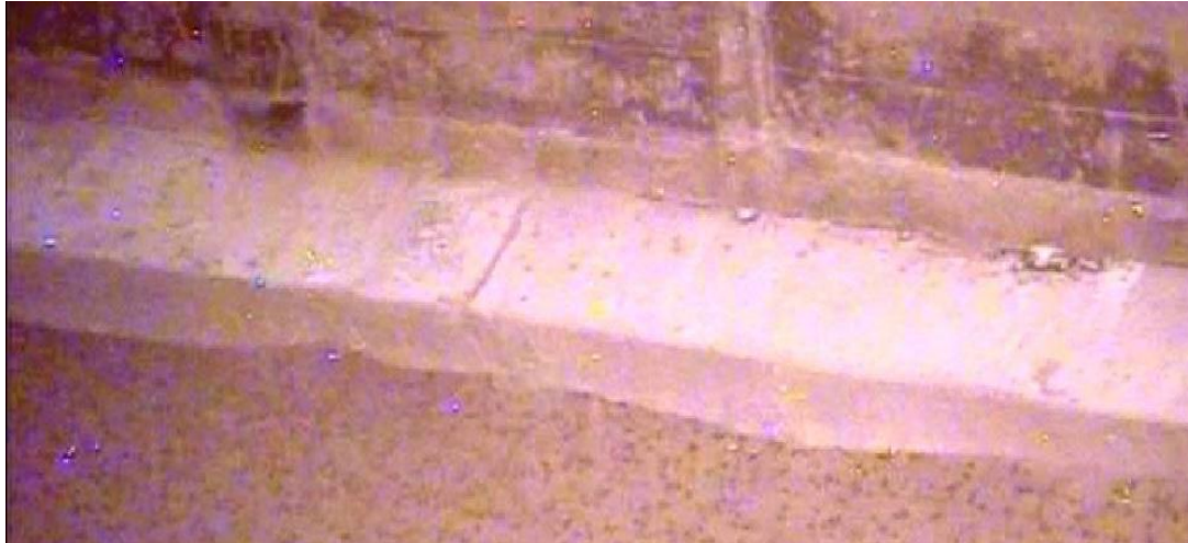
Figure 6-3: Tank 241-A-106 Steel Liner
