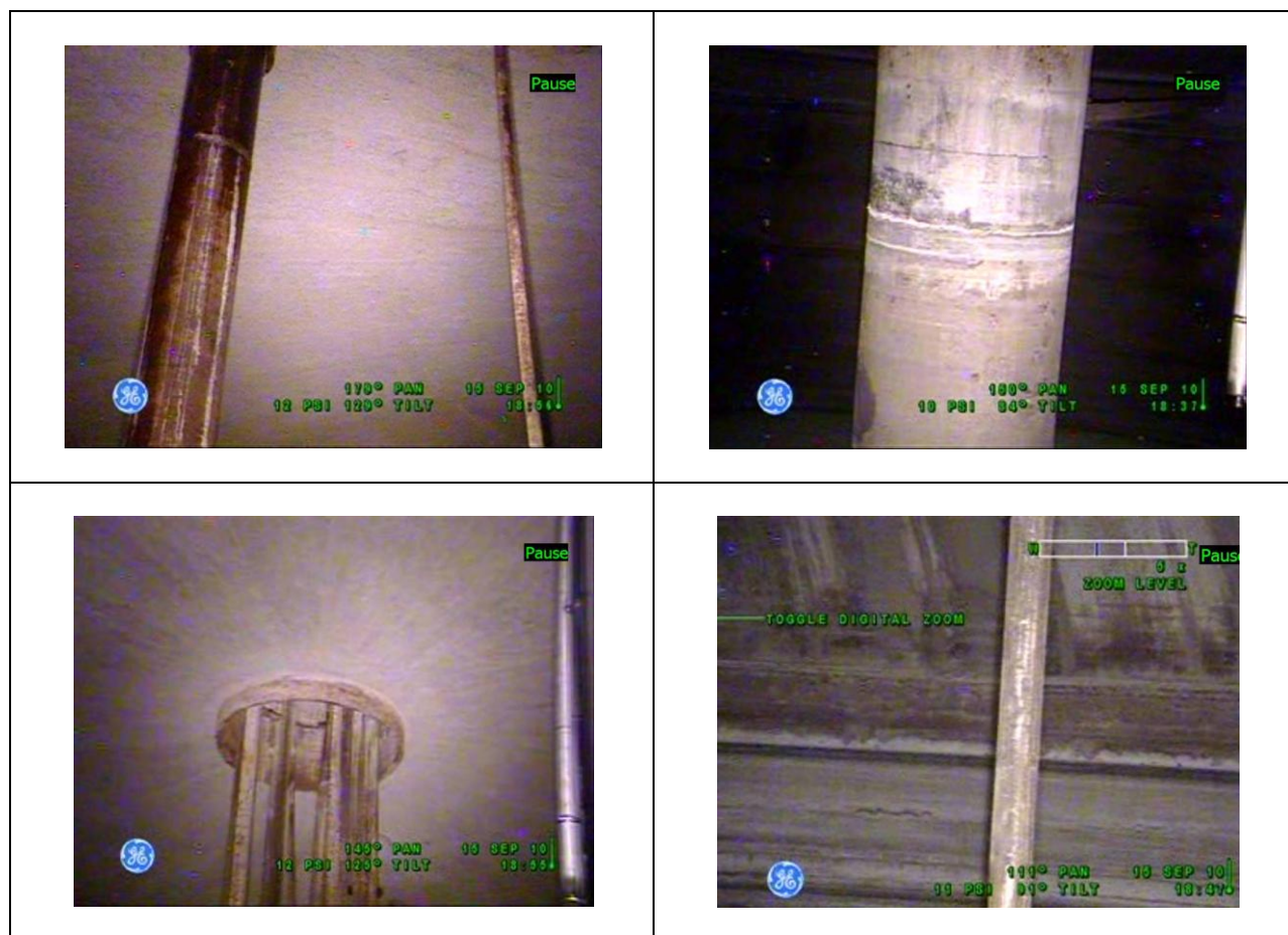
Figure 15-6: Tank 241-SX-101 In-Tank Equipment/Risers
