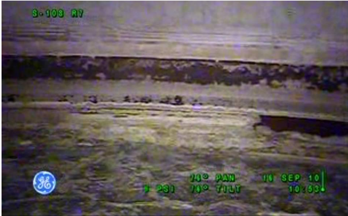
Figure 14-5: Tank 241-S-108 Steel Liner
