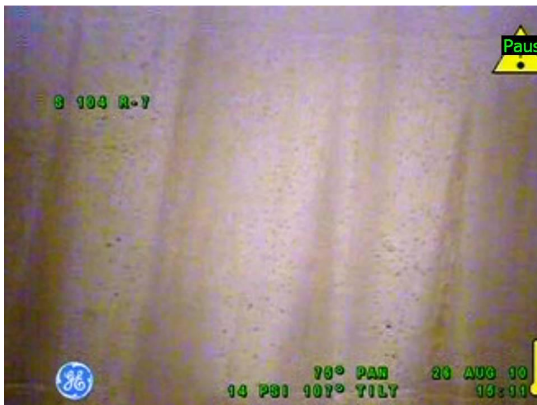
Figure 13-1: Tank 241-S-104 Concrete Dome
